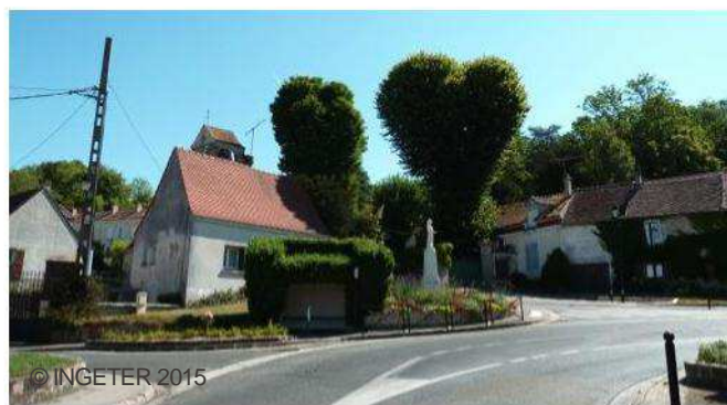
Figure 51: Square du monument aux morts.
